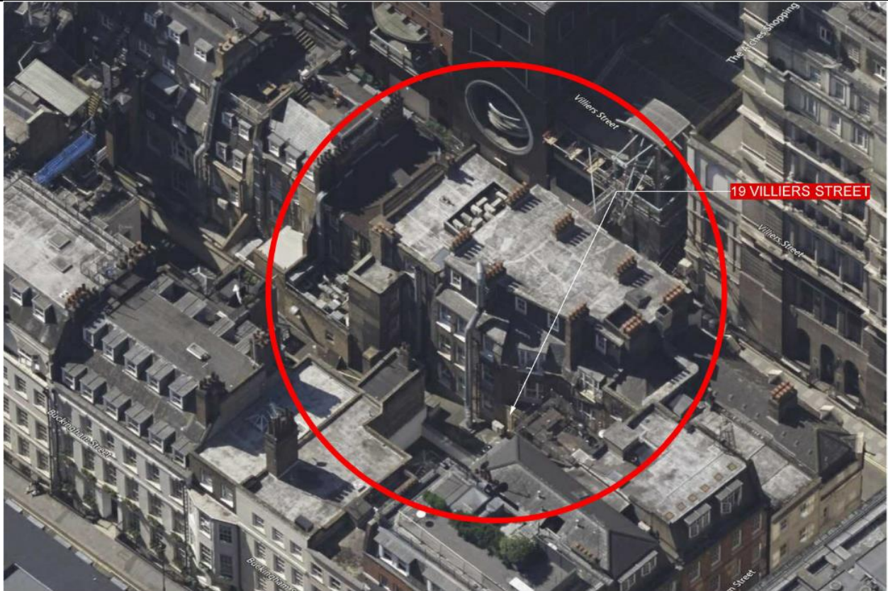
Rear of 19 Villiers Street (Aerial view)
